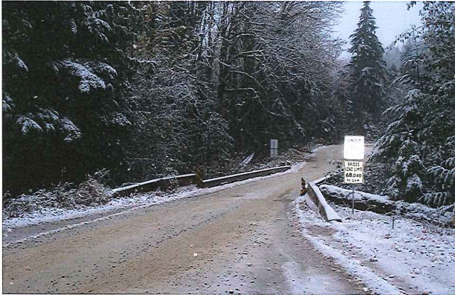
CK2129 Approach Left Bank
