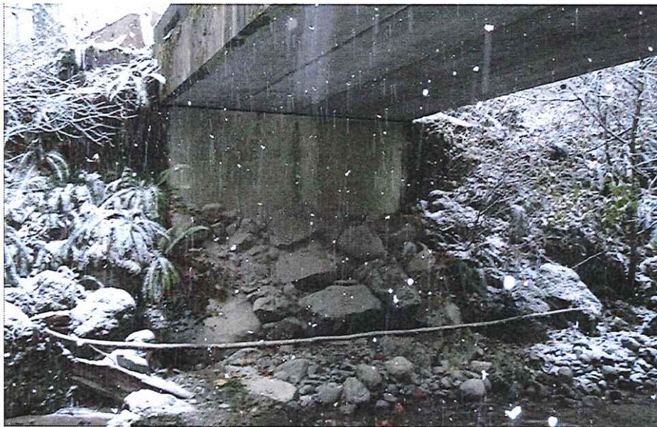
CK2129 Abutment Right Bank
