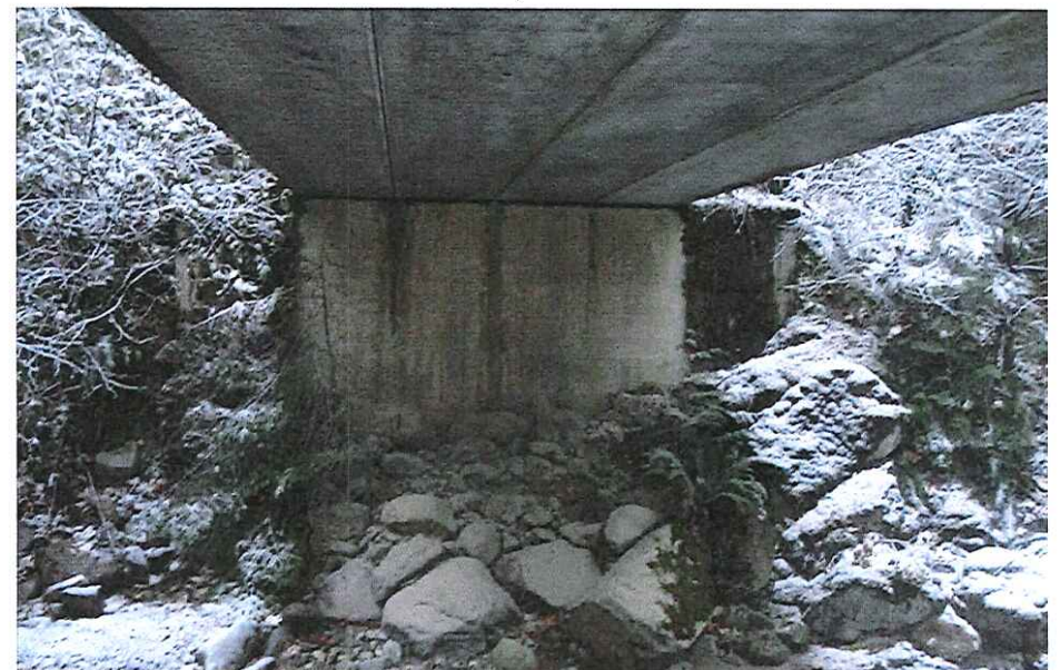
CK2129 Abutment Left Bank #2
