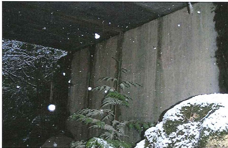
CK2129 Abutment Left Bank
